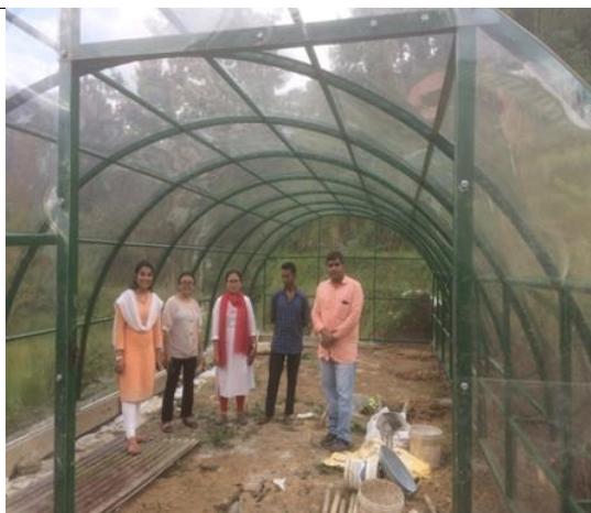
Solar dryer under construction in Soureni Assam Lingzey, East Sikkim
