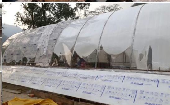
Solar Tunnel Dryer installed M/s Natures Gift, Rangpo, Sikkim
