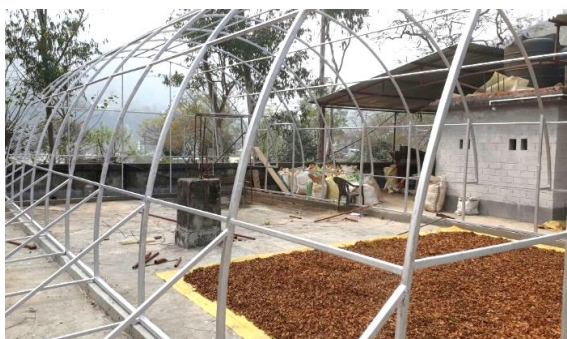
Fabricating Solar Tunnel Dryer
