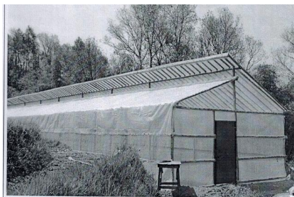
Fig. Low cost bamboo polyhouse constructed in the farmer's field
